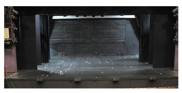
(The picture shows 88 flags, there are some more in the wings areas.) While many of the defects are smaller than the flag marking them above, others are more substantial, the largest being 70x35cm (28x14in) where water ingress occurred at a seam and lifted and distorted a larger area of vinyl.
